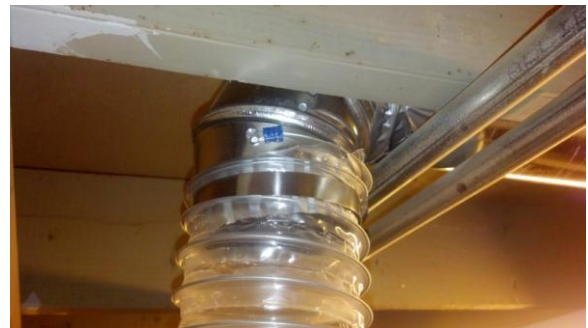
Flex hose clamped to duct and ground wire attached
