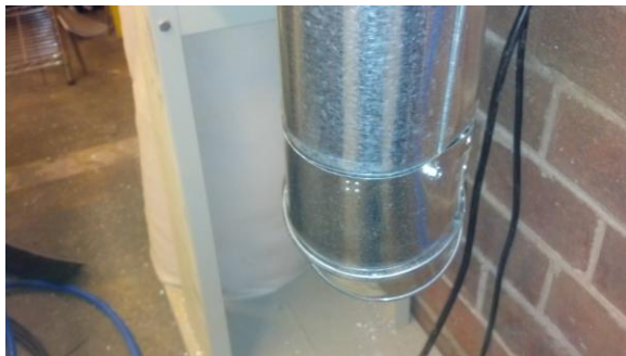
Connection screwed before taping
