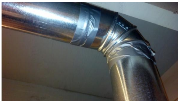
Joints Screwed and taped
