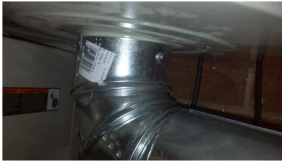
Metal Duct is screwed to collector housing with self tapping screws made for ductwork
